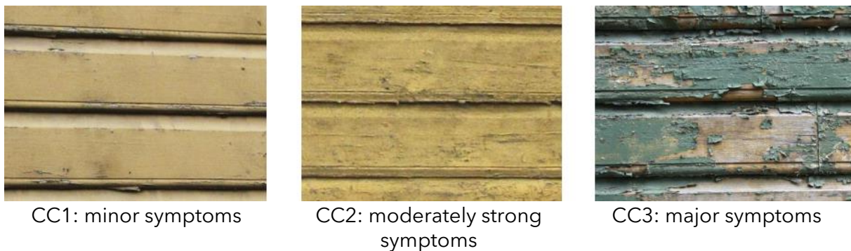
Figure 2-1: An example of condition classification of exterior paint.
