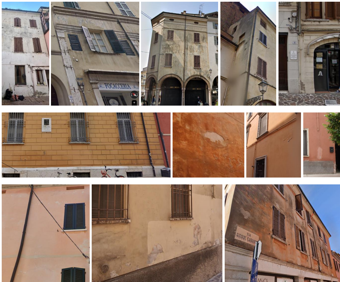
Figure 7-7 Façade photos from HeriTACE case studies and other buildings in Mantova.
