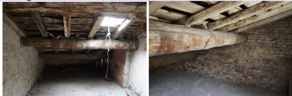
Roof construction seen from the attic - Montanara on the left, Romano on the right
